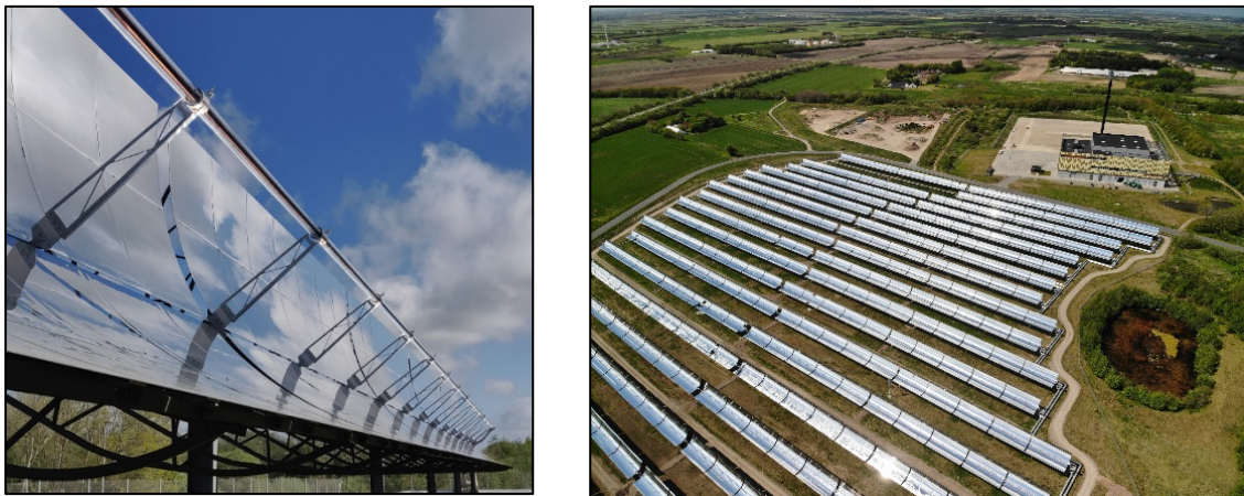
Figure 2: Left: Close up photo of the parabolic trough collector mirrors and receiver tube. Right: Aerial photo of the solar collector field and power plant in the background.
